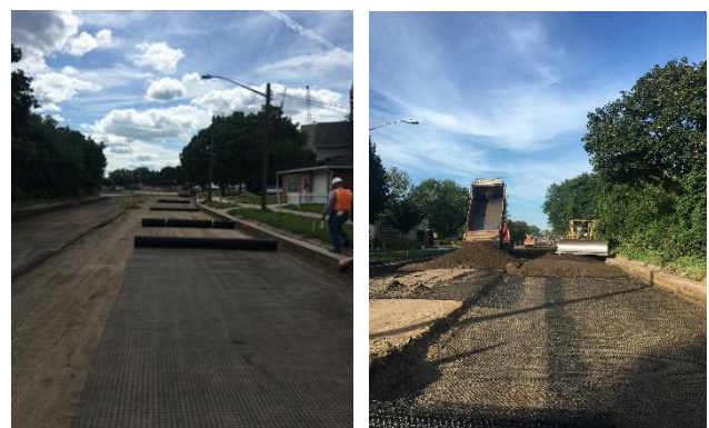
a) Laying out geogrid b) Placing base course materials
