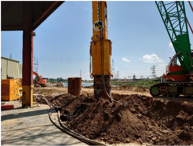
Figure 11. Driving 1400mm diameter piles with hydraulic impact hammer
