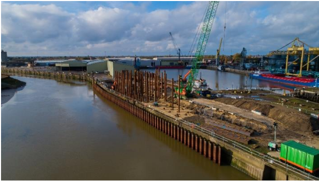
Figure 10. Left bank during construction
