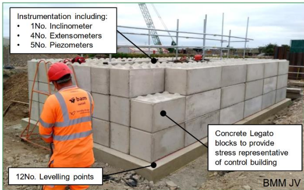
Figure 6. Large scale load test – completed height monitored for 10 days
