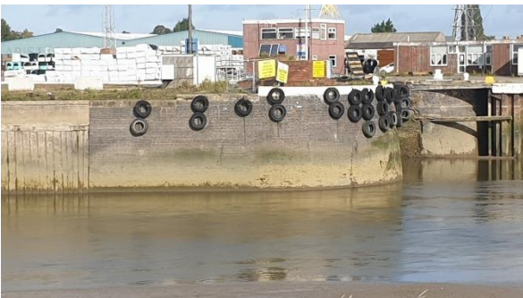
Figure 15. Southern elevation of the existing knuckle
