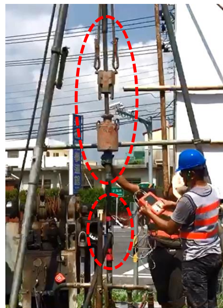
Figure 6. Auto-drop hammer system and hammer energy inspection arrangement adopted in the Phase I soil liquefaction study in Huwei & Tuku Township, Yunlin County, Taiwan.
