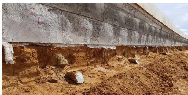
Figure 11. Site photo on the cave-in of the exposed sand layer
