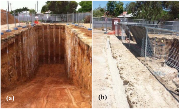
Figure 2. (a) Trial pit of up to 8m depth, (b) Trench for application of water at the trial
