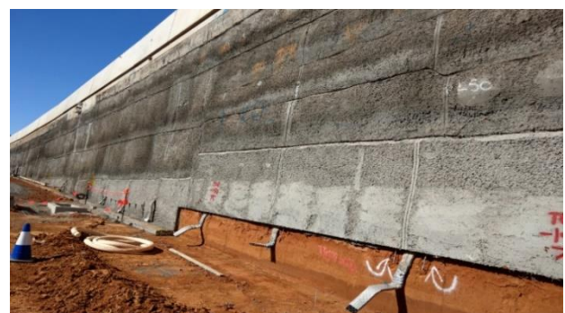
Figure 18. Soil nail wall after full depth excavation
