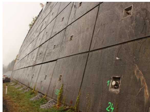
Figure 1. Anchored retaining structure along an Austrian highway
