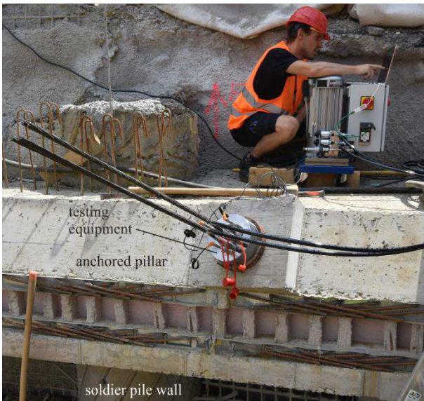
Figure 9. Field Testing of the developed anchor test equipment
