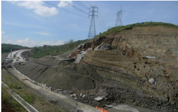
Figure 1. Slope failure on clay shale at STA 19+250 Semarang-Bawen tol road during construction (Himawan 2013)
