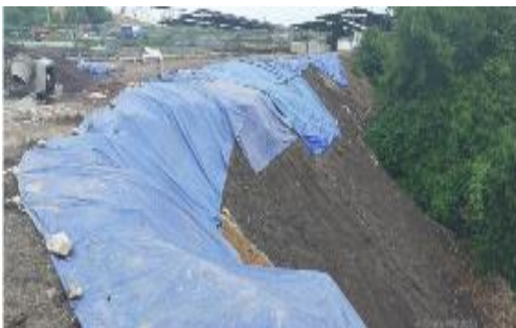
Figure 2. Slope are backfilled with weathered argillaceous rock at Cariu, West Java, Indonesia, before failure on Januari 21 th , 2020 (Alatas 2020)
