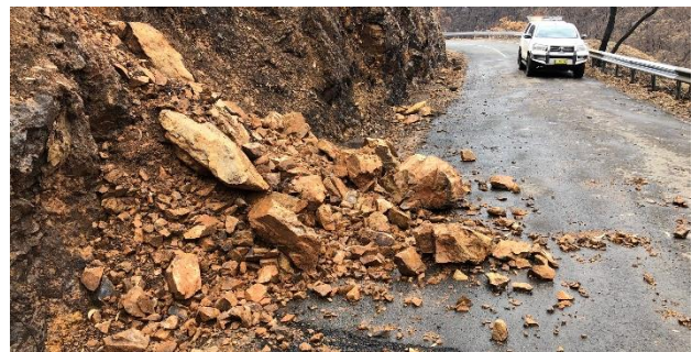
Figure 11. An approximately 4m 3 wedge failure resulting in broken interbedded siltstone and sandstone fragments comprising gravel, cobbles and boulders up to 800mm across.
