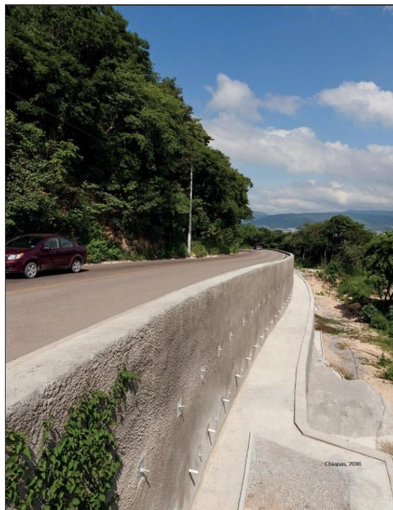
Figure 1. Slope Stabilization with Estatec System with two levels in mountain areas in Chiapas (México).
