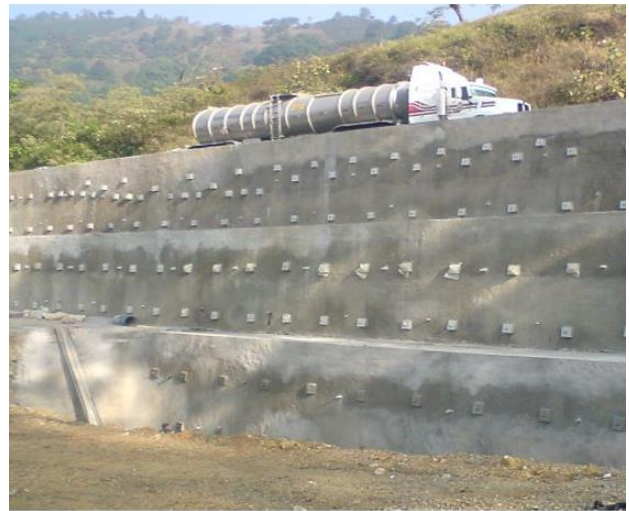
Figure 3. Pachuca – Tuxpan Road, Km 105+200. 3 levels Estatec
