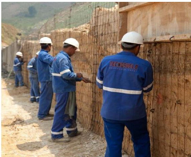
Figure 15. Preparation of cement-bentonite wall for shotcrete
