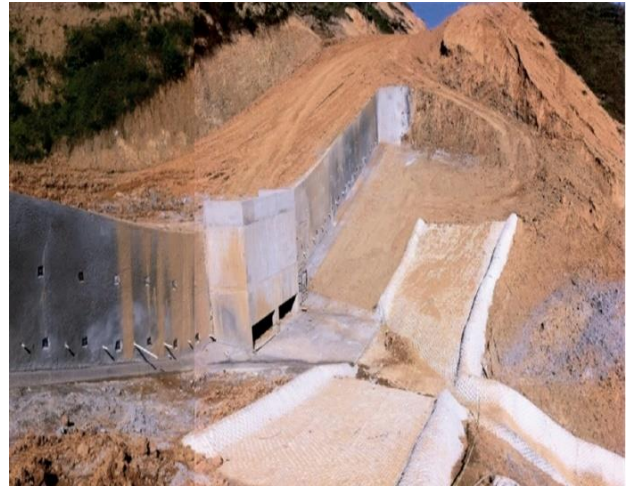
Figure 7. Km 2+600 Zoquital – Catalina pipeline. One level Estatec and erosion protection system.
