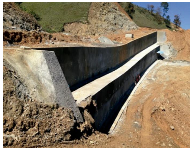
Figure 5. Km 2+720 Zoquital – Catalina pipeline. Stabilization with Estatec System.
