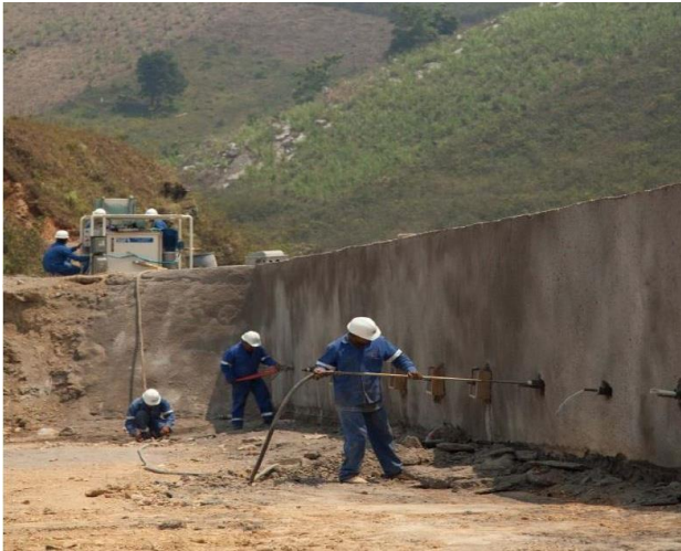
Figure 14. Grouting of soil improvement in active and passive nails.
