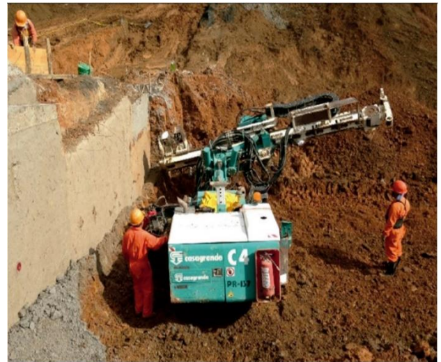
Figure 13. Drilling of nails.
