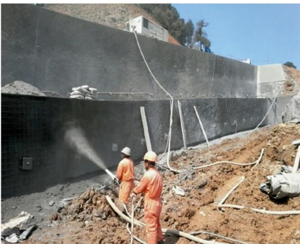
Figure 16. Shotcrete on cement-bentonite wall parament.
