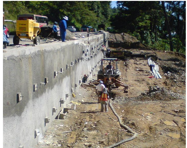
Figure 12. Excavation of cement-bentonite wall with conventional machinery.
