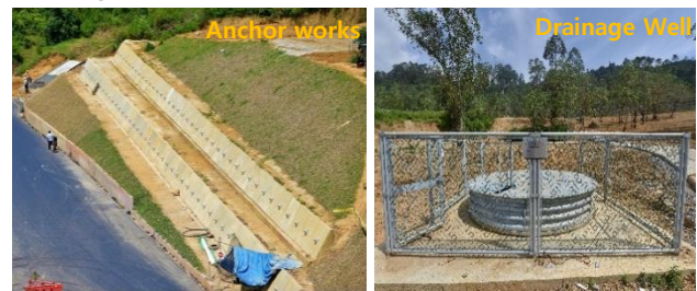
Figure 13. Photographs of implemented countermeasures
