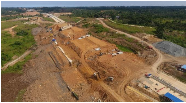
Figure 11. Progress of soil reinforcing using bored pile, PC piles and berm
