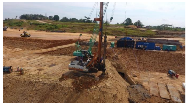
Figure 10. Bored piles construction
