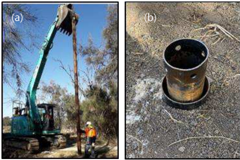
Figure 4. Photos of (a) pile installation; and (b) installed pile.
