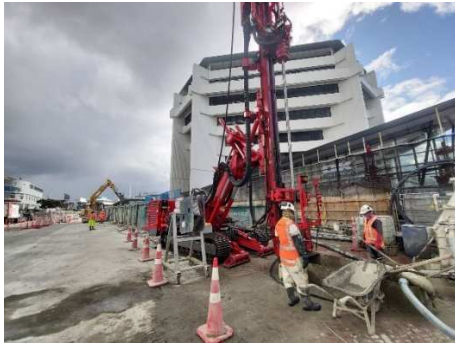
Figure 3: Execution of jet grouting columns on site.
