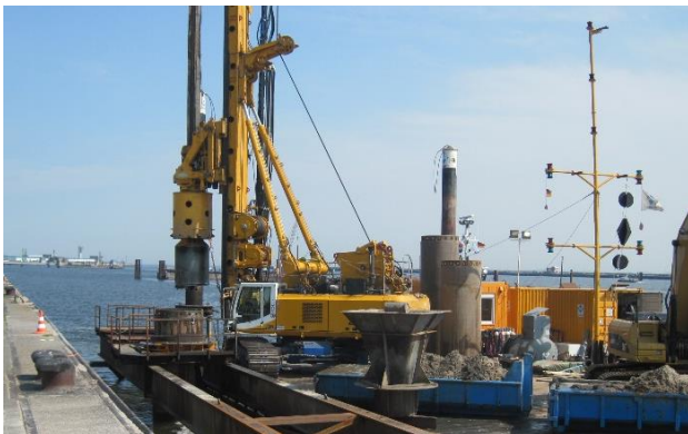
Figure 3. Execution of the soils exchange drillings
