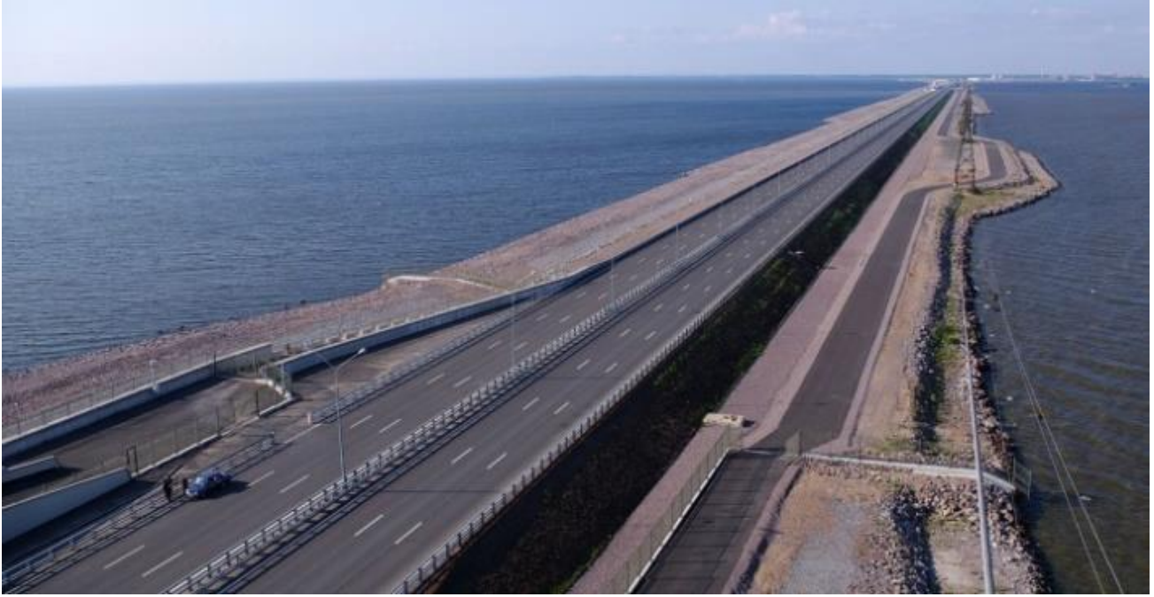
Figure 4. A view of the current state of the high-speed highway on the Complex of Structures of the City of St. Petersburg from Floods
