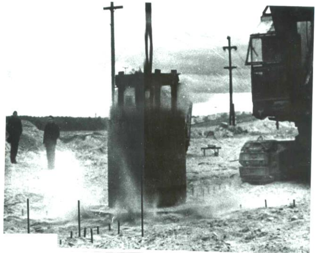
Figure 2. The moment of dropping the experimental variant of a heavy dual mass tamper
