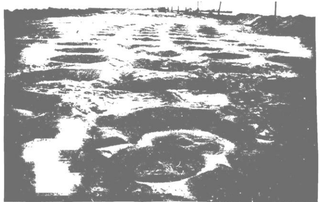
Figure 3. The general view of the foundation site after being treated with the designed variant of a dual mass tamper with a view of soil settlements under its sole
