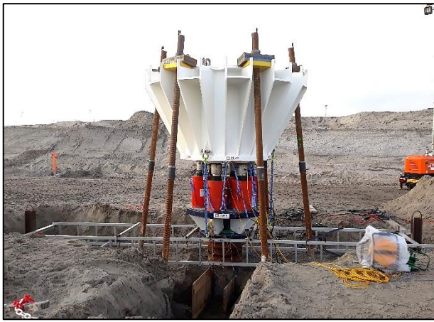
Figure 3. Pile test frame and the reaction anchors used at the Maasvlakte test site
