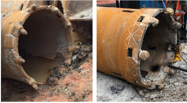
Figure 5. Rock Coring / Excavation tools: Core barrel.
