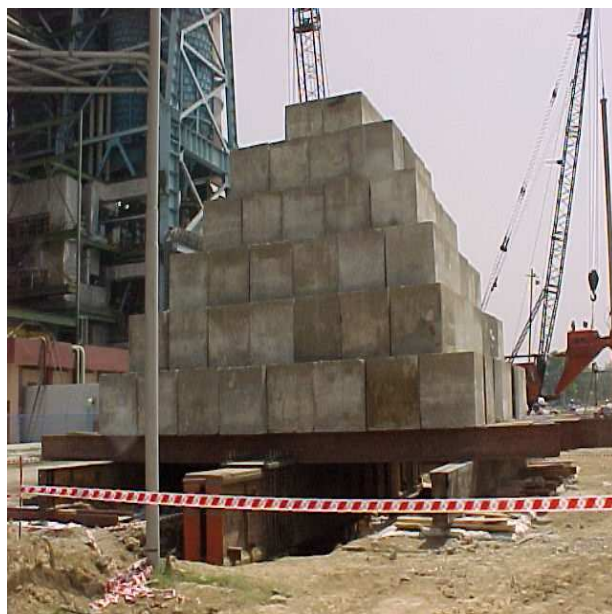
Fig 3 Typical platform and kentledge for initial pile load test.
