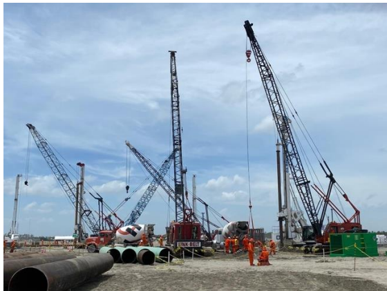
Figure 3. Overview of drilled shafts construction.
