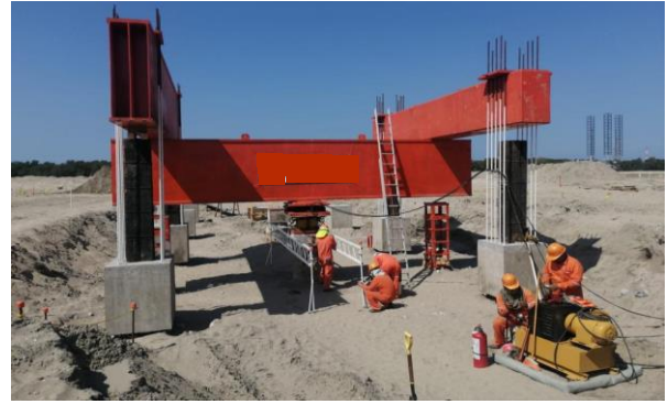
Figure 4. General arrangement for compression static load test.
