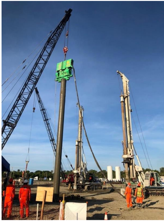
Figure 2. Steel casing placement with vibrodriver.
