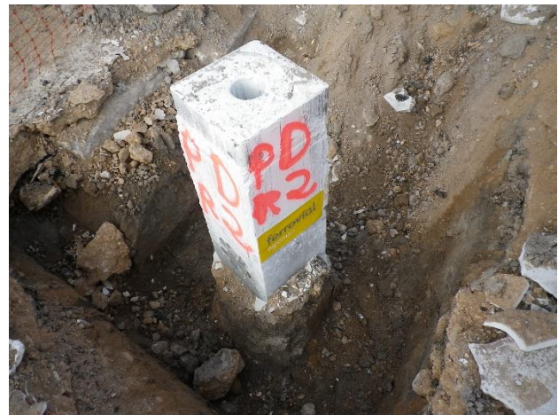
Figure 12. Excavated shaft grouted driven concrete pile
