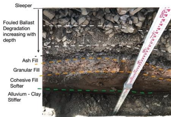
Figure 1. Typical soil profile (perpendicular to existing track alignment) recorded during N2NS geotechnical investigation showing typical 'w' shaped (orange dash), ash and progressive ballast degradation.
