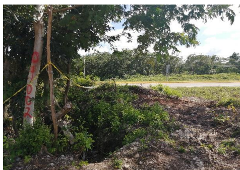
Figure 1. (a) An old embankment in Yucatan, (b) a sinkhole next to the old embankment and (c) a sinkhole next to the road at 1.5km from the previous sinkhole.
