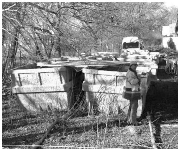
Figure 10. Transport skips as backwash storage. They had to remain on site for over a month.
