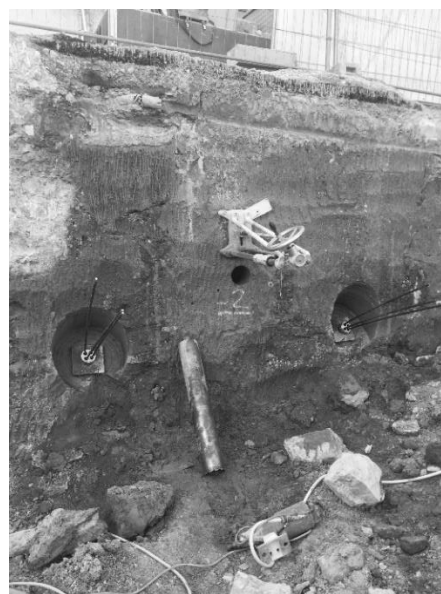
Figure 9. Core drilling being taken from the jet grouting wall at the Rittergasse site. The upper level at -2.0m bGL is shown. The location is directly below the eastern washing machine as shown in Figure 7.
