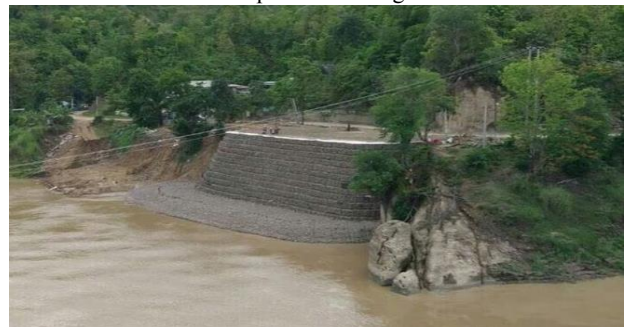
Figure 3. Trial wall after construction.
