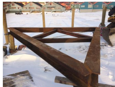
b) Triangular-shape footing setup
