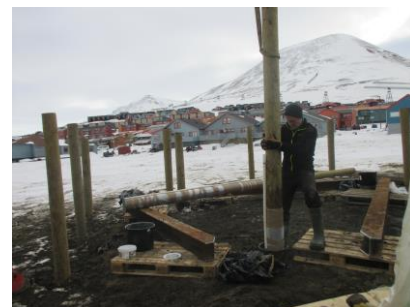
a) Footing pile installation
