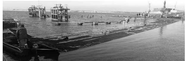
Figure 2. Geotube placement at the Ancona CDF.
