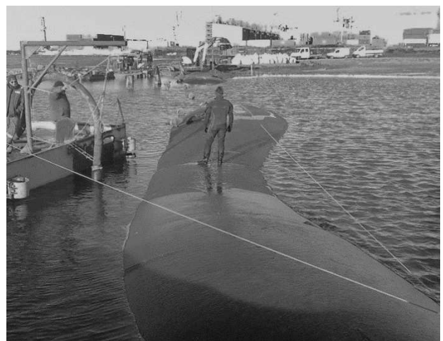
Figure 4. Filling phase of the geotube at the Ancona CDF.
