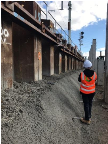
Figure 4. Temporary sheet pile wall portion supported by soil nails and buttressed with berm at the piling platform level. Prisms installed at wall top and mid-height for displacement monitoring.
