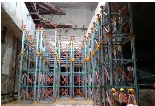
Figure 14. Vertical props provided to construct the retrieval platform for the upper TBM arriving at the Southern end.
