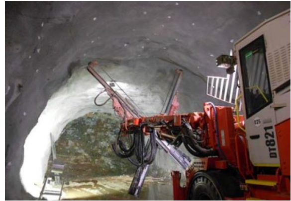
Figure 6 - Drilling for the installation of the tiles (MDR, 2019).
