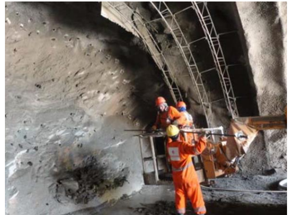
Figure 7. Installation of metal camats in the tunnel entrance (MDR, 2019).
