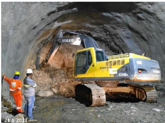
Figure 4. Removal of loose blocks in front of tunnel excavation (MDR, 2019).
