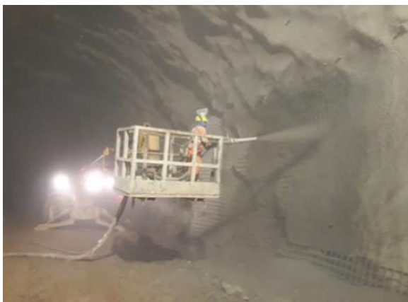
Figure 5. Application of projected concrete on walls and vaults (MDR, 2019).
