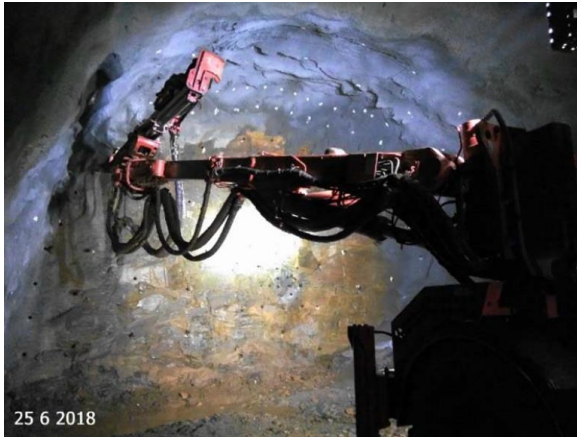
Figure 3. Excavation cycle with drilling of the tunnel fire plane (MDR, 2019).
