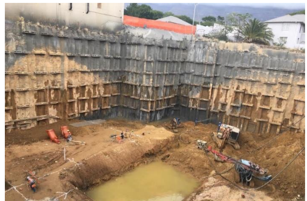
Figure 2. Photo of Deep Excavation, Gardens, Cape Town
