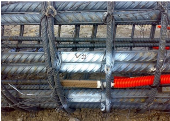
Figure 7. Quarter-bridge strain gauge attached to the steel reinforcement.
