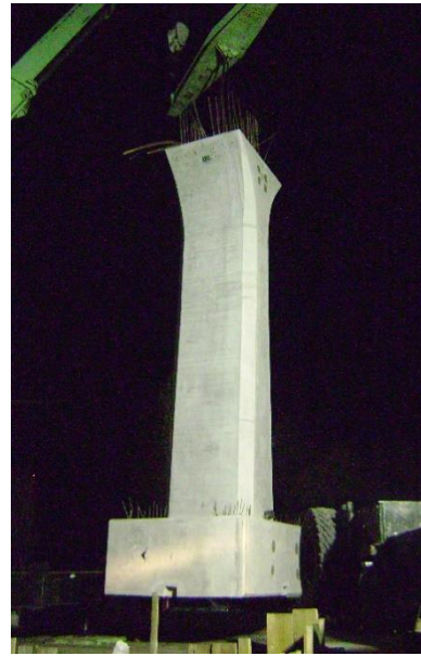
Figure 3. Mounting the footing-column unit during the early morning.
