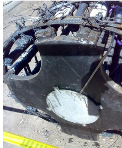
Figure 8. Installing the pressure cell at the tip of the steel reinforcement of pier 4.
