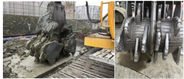
Figure 4. Cutter Soil Mixing Head and Operating Rig
