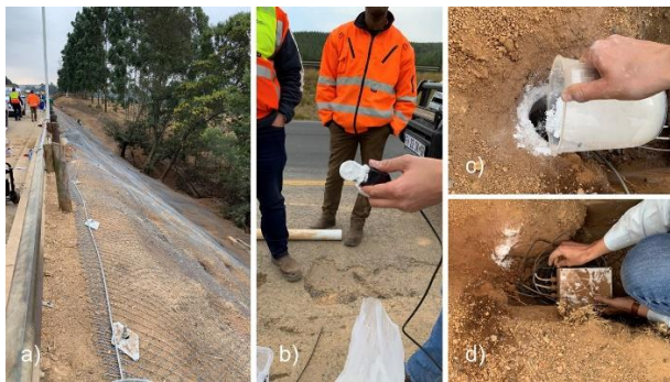
Figure 5. System installation (a) Site overview with DAQ located at white standpipe, (b) Teros 21 sensor coated in silica flour, (c) pouring premeasured volume of silica flour down borehole and, (d) DAQ placed beside filled in borehole.
