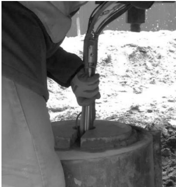
Figure 4. VWSG Model 1300 A-9 installation in a pile.
