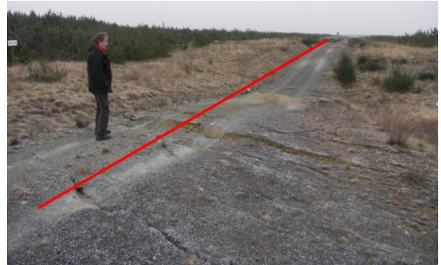
Figure 3. Surface collapse (path originally running horizontally, red line) at the former Schlabendorf-South open-cast mine.
