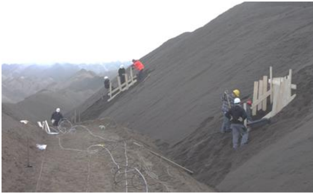
Figure 6. Installation of stress measuring stations and cross-bedding of dump.
