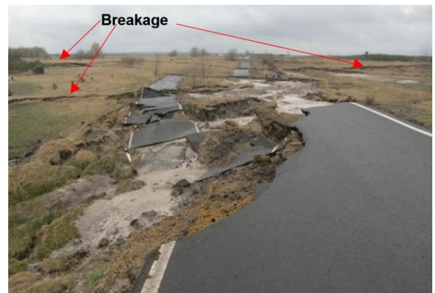
Figure 5. Flow liquefaction with breakages at former Schlabendorf-South open-cast mine in 2008.
