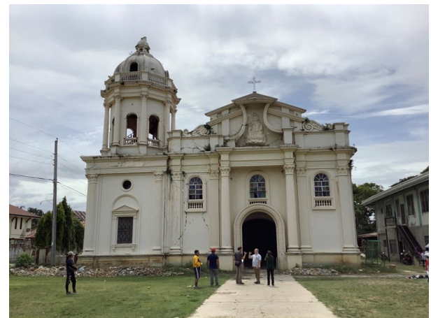
Figure 2. The façade of the Antequera Church showing structural damage after the major Bohol 2013 earthquake.
