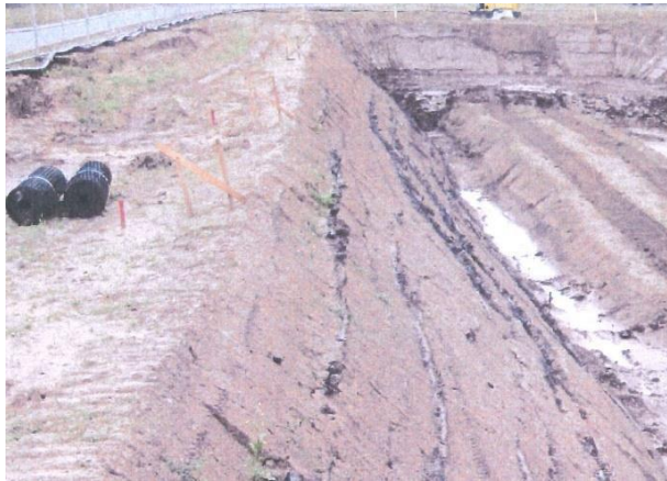
Figure 7. View of back-scarp and toe bulge.
