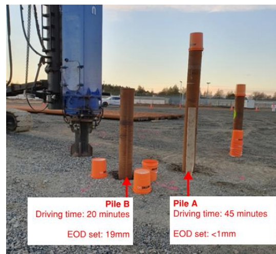
Figure 5. Set-up verification test
