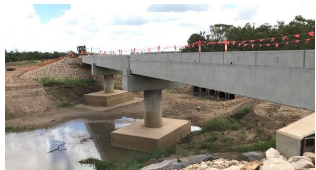
Figure 1. View of completed bridge from case study.
