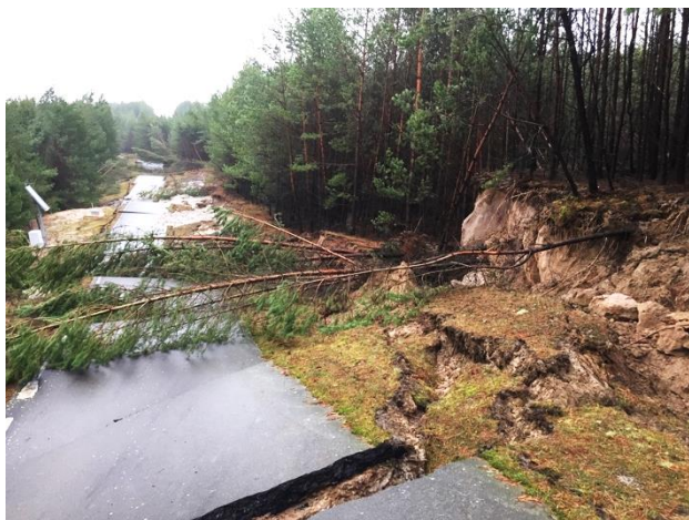
Figure 1. Consequences of the soil liquefaction event of 18.12.2017 in the former Schlabendorf-Süd open pit, photo of 21.12.2017.
