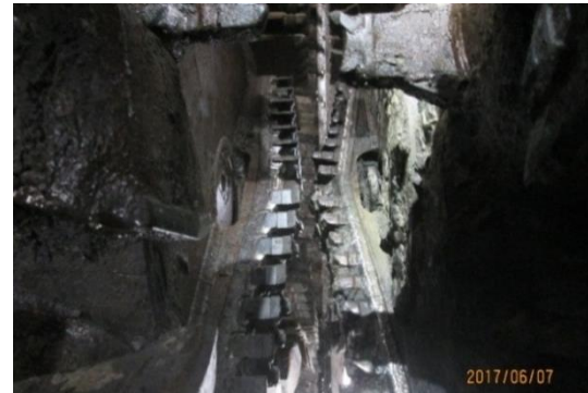
Figure 5. Two TBMs docked together
