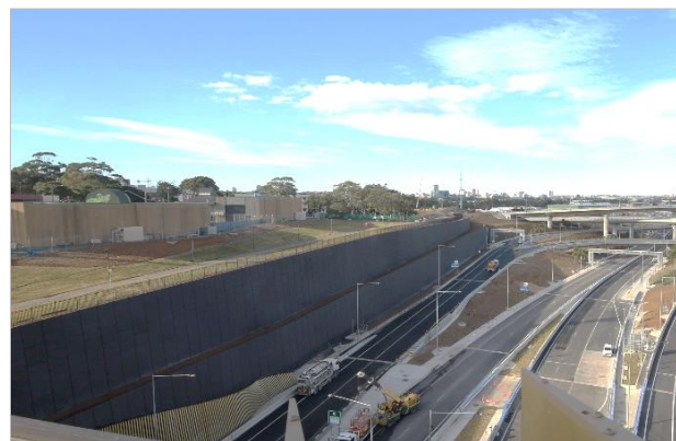
Figure 13. Completed RSW.
