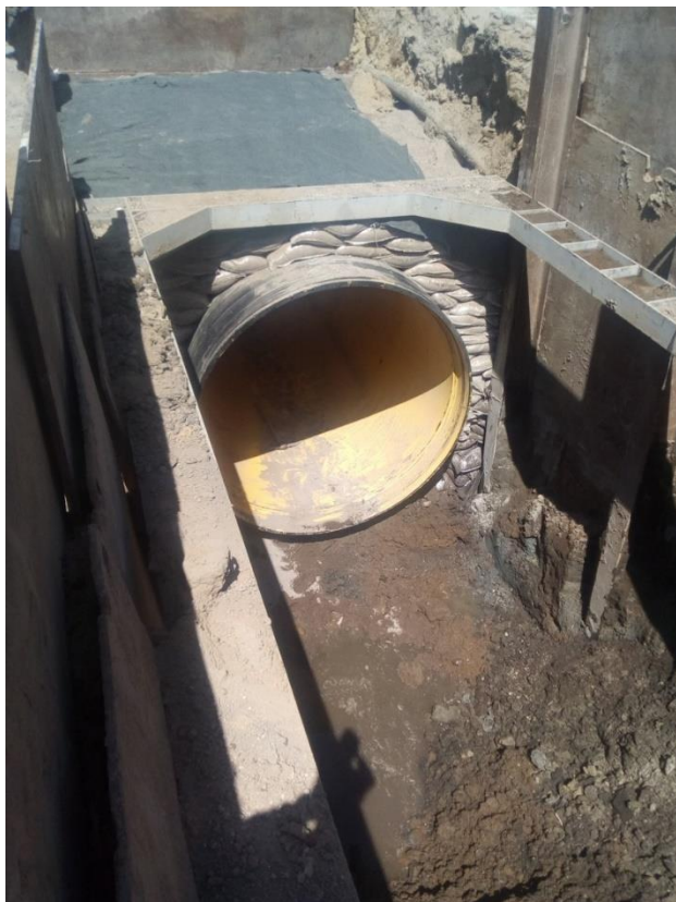
Figure 22. Protection of culvert in area affected by soil cracks.
