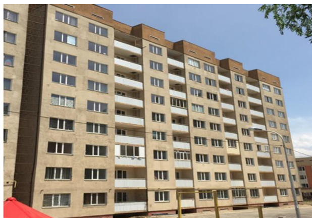
Figure 18. Tilted RC Apartment House with 9 stories (Bespaev,2019)
