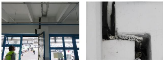
Figure 3. Uncoupling of structural elements.
