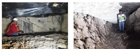
Figure 5. Loss of contact between the raft and the ground.
