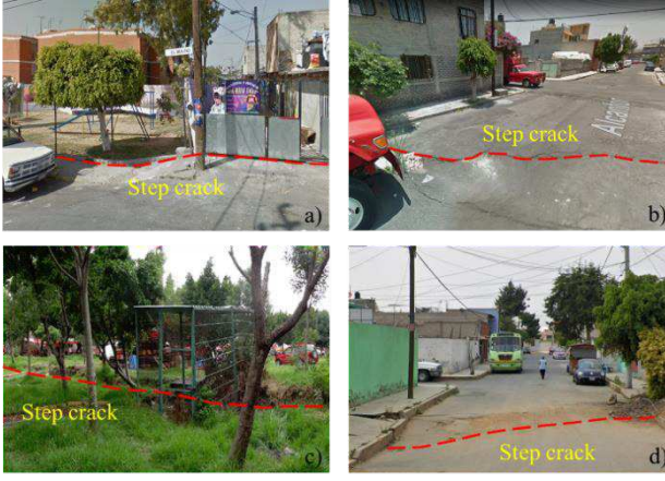
Figure 2. Step-shaped cracks in the study sites
