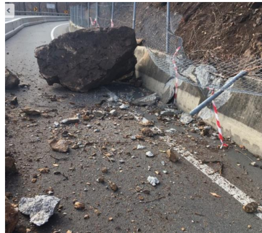
Photo 2: Boulder crash through concrete barrier into closed uphill lane following 23 mm / 24 hours rainfall event of 26 December 2019 (source: TMR)
