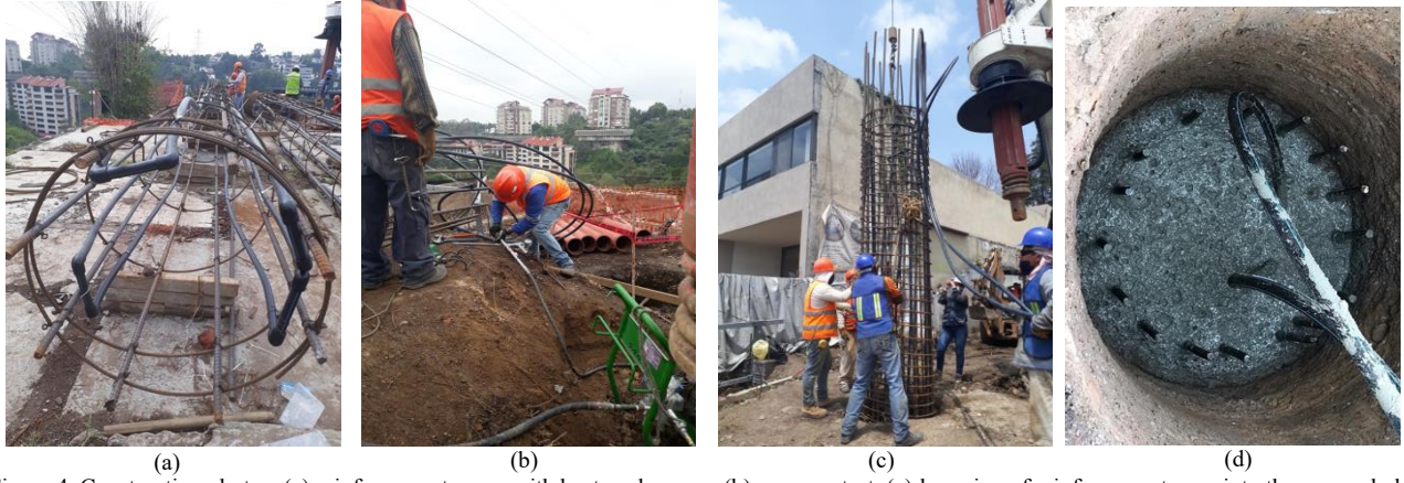
Figure 4. Construction photos: (a) reinforcement cages with heat exchangers, (b) pressure test, (c) lowering of reinforcement cage into the uncased hole, and (d) concrete pouring.
