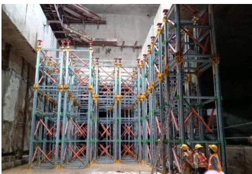
Figure 14. Vertical props provided to construct the retrieval platform for the upper TBM arriving at the Southern end.
