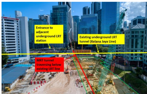
Figure 1. Ampang Park Station Site
