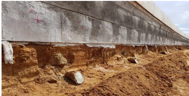
Figure 15. Site photo on the cave-in of the exposed sand layer
