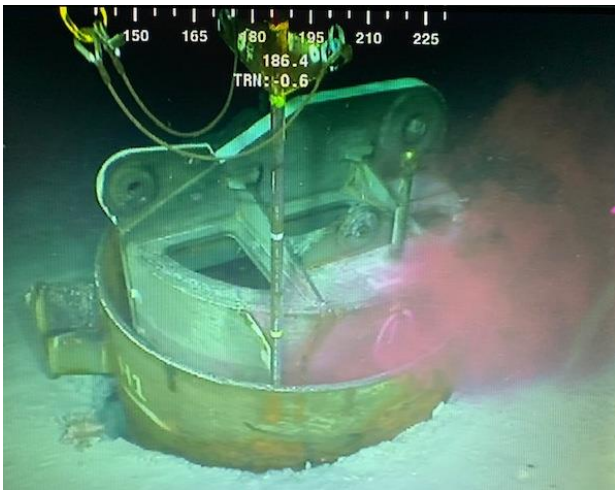
Figure 12. Grouting operations – observing visual marker released by stinger at pile base to check obstructions are not present
