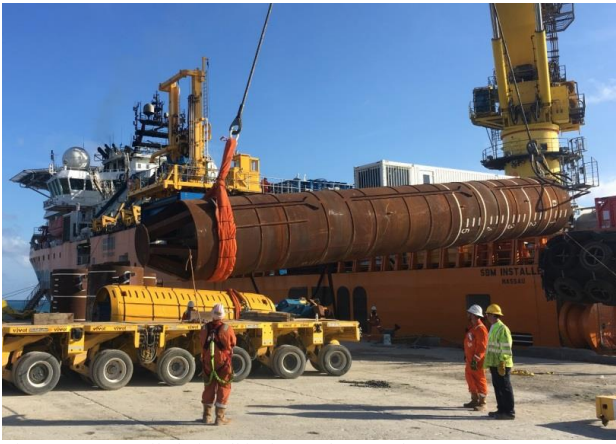
Figure 7. Insert pile being lifted onto the vessel
